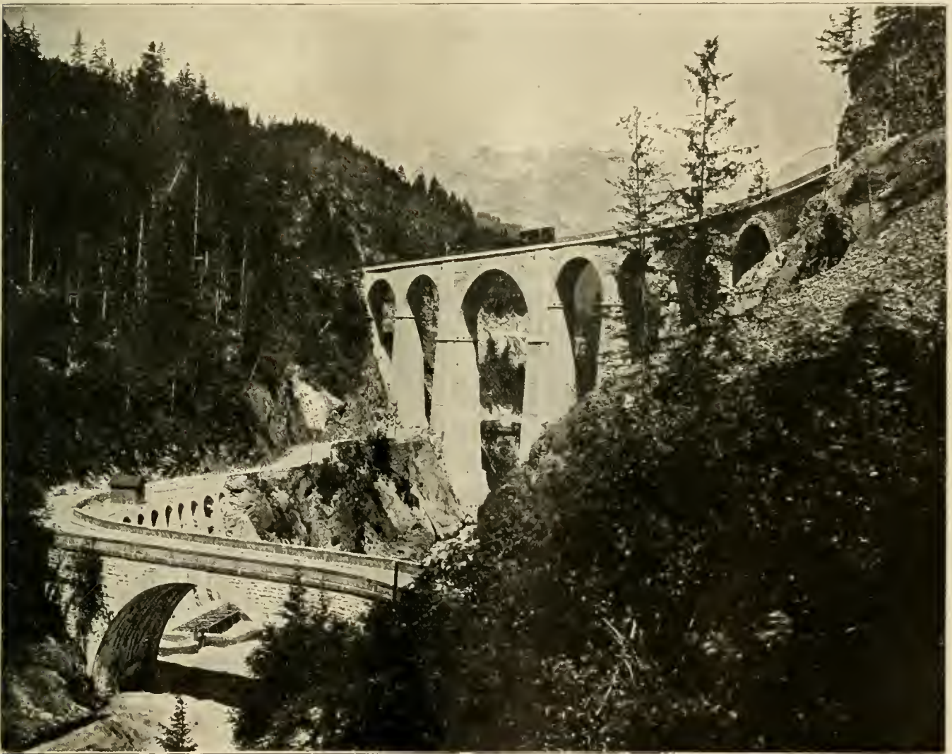
VIADUCT SAINTE MARIE ON CHAMONIX RAILWAY, SWITZERLAND.
